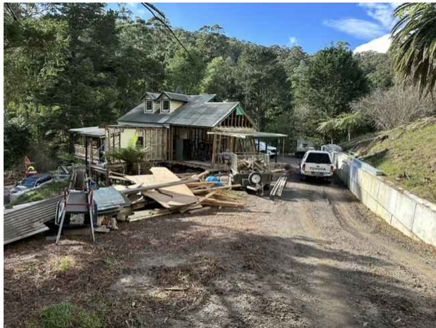
AREA 7 DRIVEWAY & FLAT PAD FOR HOUSE PARKING
